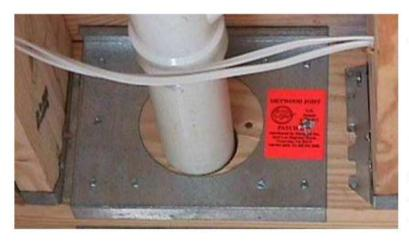
Use the 2810HR Joist Reinforcer to allow placement of up to 6" holes in 2x10 wood joists and 4 ½" holes in 2x8's. The 2810HR Reinforcer comes to you in 2 identical pieces, which are simultaneously attached to a joist to accommodate a hole in the joist which may have pipes, conduit, wires, etc., already in place.
